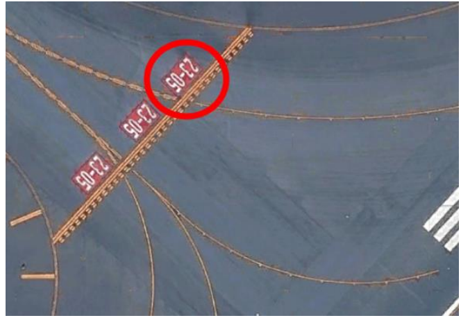
<Photo 2: Surface paint requiring consideration for removal>
